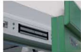
electromagnetic lock with counterplate surface-mounted
